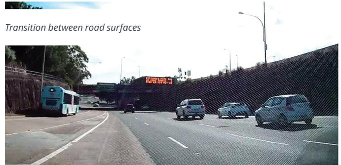
It appeared that the difference in contrast between these road surfaces interfered with lane keeping systems, either leading vehicles out of their lane, or disengaging lane keeping.
